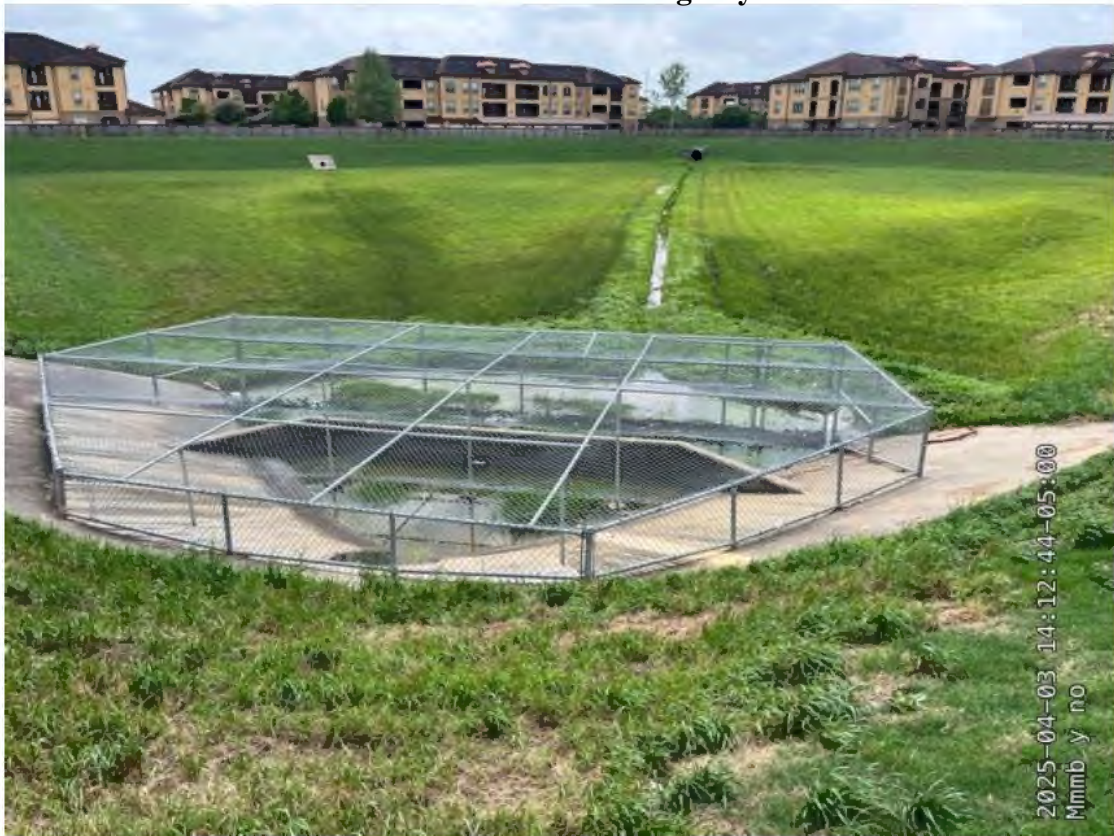
East Pond – Wash Out @ Emergency outfall
