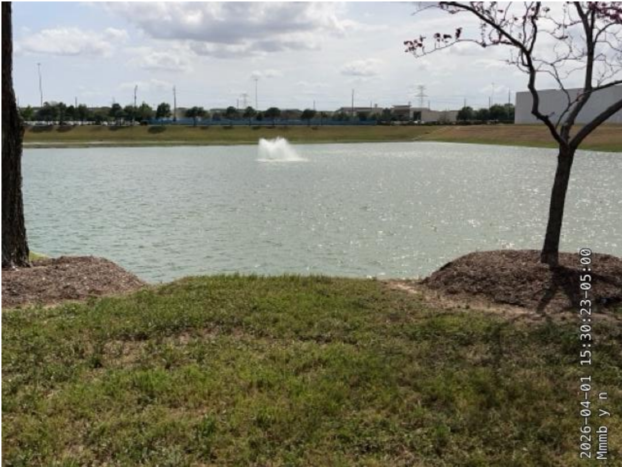
Mason Creek Detention Pond
